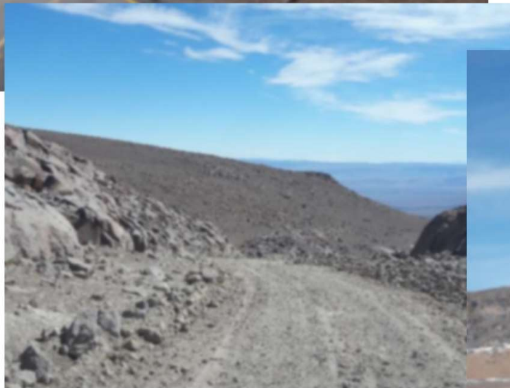
Internal roads At km 35
